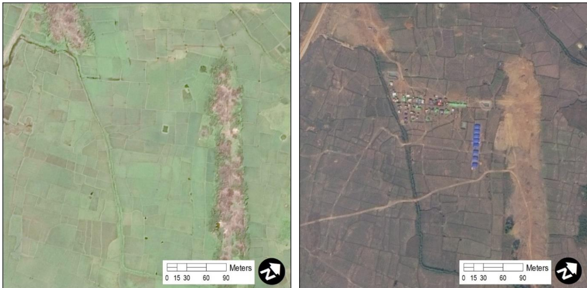
Figure 15: Terrain clearance and new construction at Inn Dinn (Middle) village, Maungdaw Township
